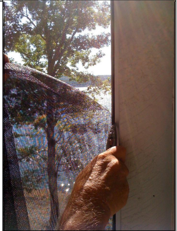
**21. TUCK SPLINE INTO CORNERS USING THE TIP OF A SCREWDRIVER.**
