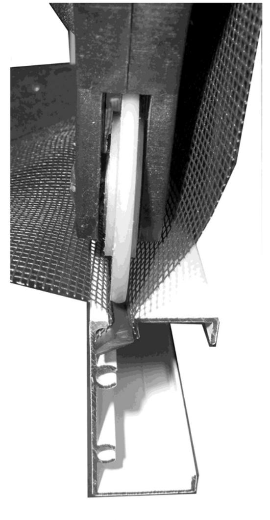
15. MEASURE SIDE (A) AND CUT OFF PIECE OF SPLINE 6" LONGER.
