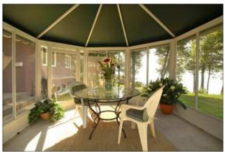
• These specialty spa enclosures have a **Roof Structure** that is made of 1.5" square extruded aluminum with a baked on enamel finish. Once up, there is no need to take it down!
