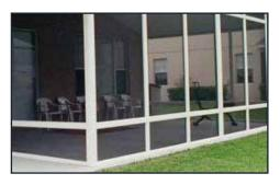
Horizontal chair rails are recommended if you don't have a kick plate and your openings are larger than 54". They can be placed at any height. We recommend somewhere below the midpoint to create a clear line of sight for when you are seated in the room.
