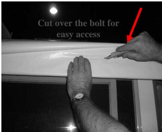
slit in the Fabreen® to access the bolts which will tension the system. There are 3 bolts per system, on each side and in the middle.
